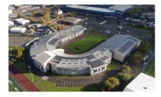
Kembla supplied and installed a 304.85kWp system maximising the curved roof on the building. The existing plant room provided perfect conditions for the installation.
